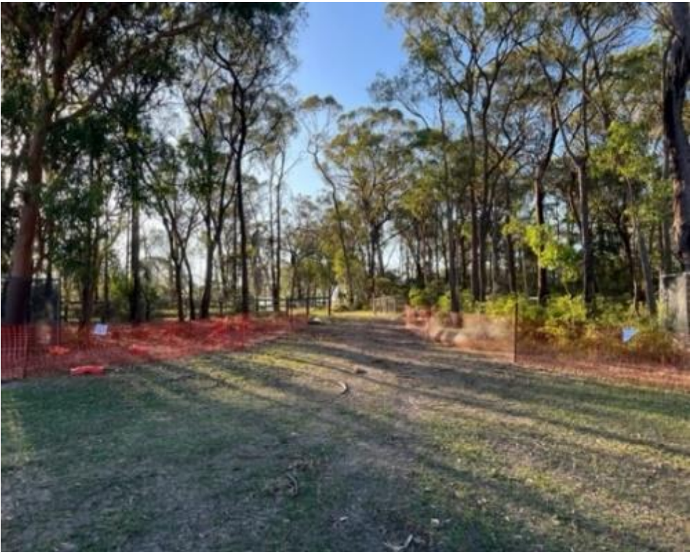
Figure 11 – Tree protection fencing
