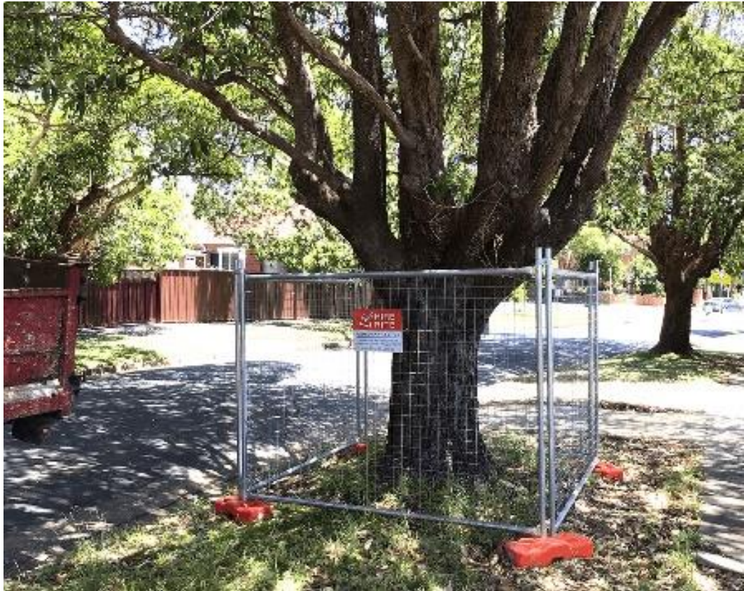
Figure 12 – Examples of tree protection fencing
