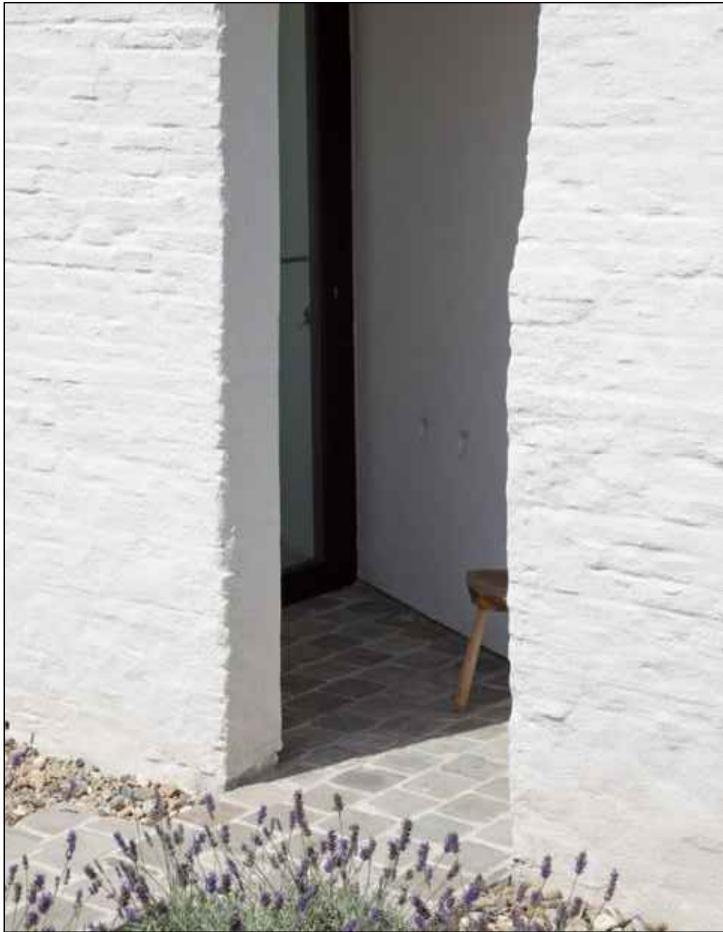
example of rough bagged and painted exist split block piers in 'Lexicon Quarter' paint colour
