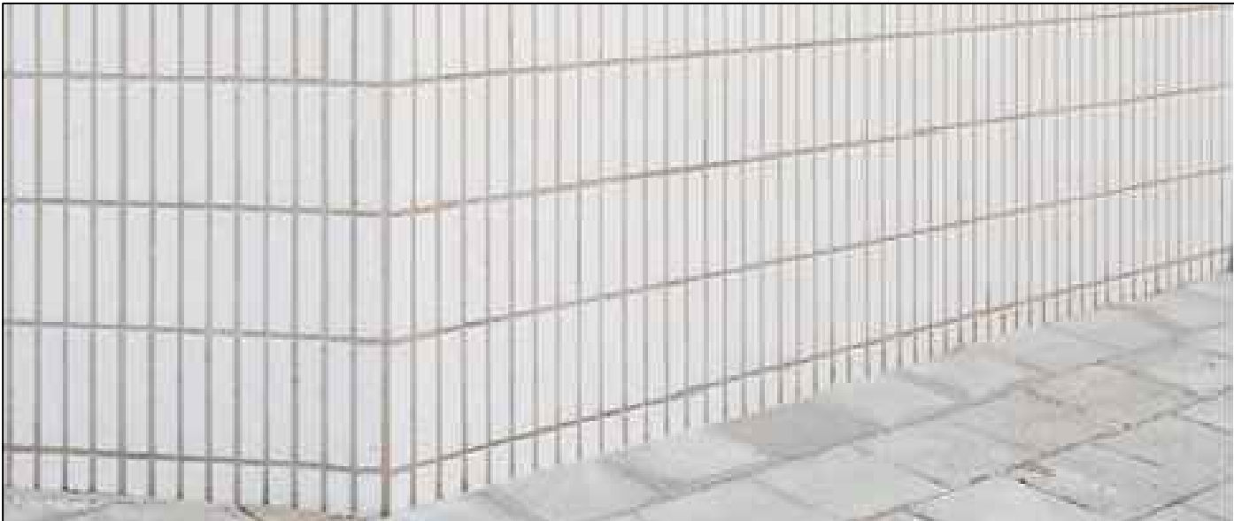
vitrified white wall tile (ie 80x240) to inside and outside face of rc up-stand element of balustrade on upper deck - and the proposed stack bond look in context
