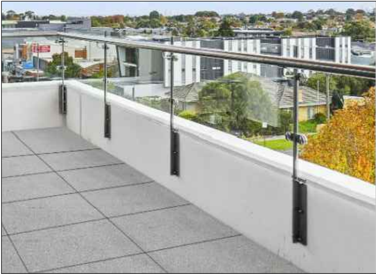
example of proposed frameless glass balustrade with integrated ss tubular handrail and fixing arrangement (balcony upstand however to be tiled)
