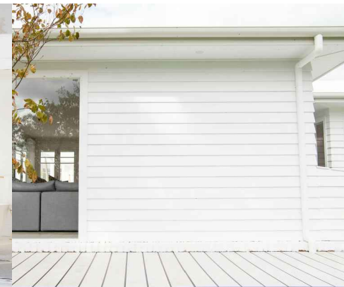
CL1 WHITE WEATHERBOARD CLADDING
