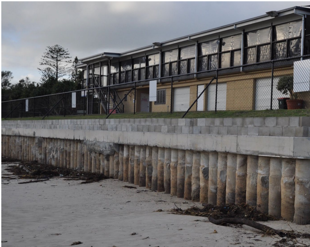
Photo of Kingscliff SLSC Secant wall (Gordon)
