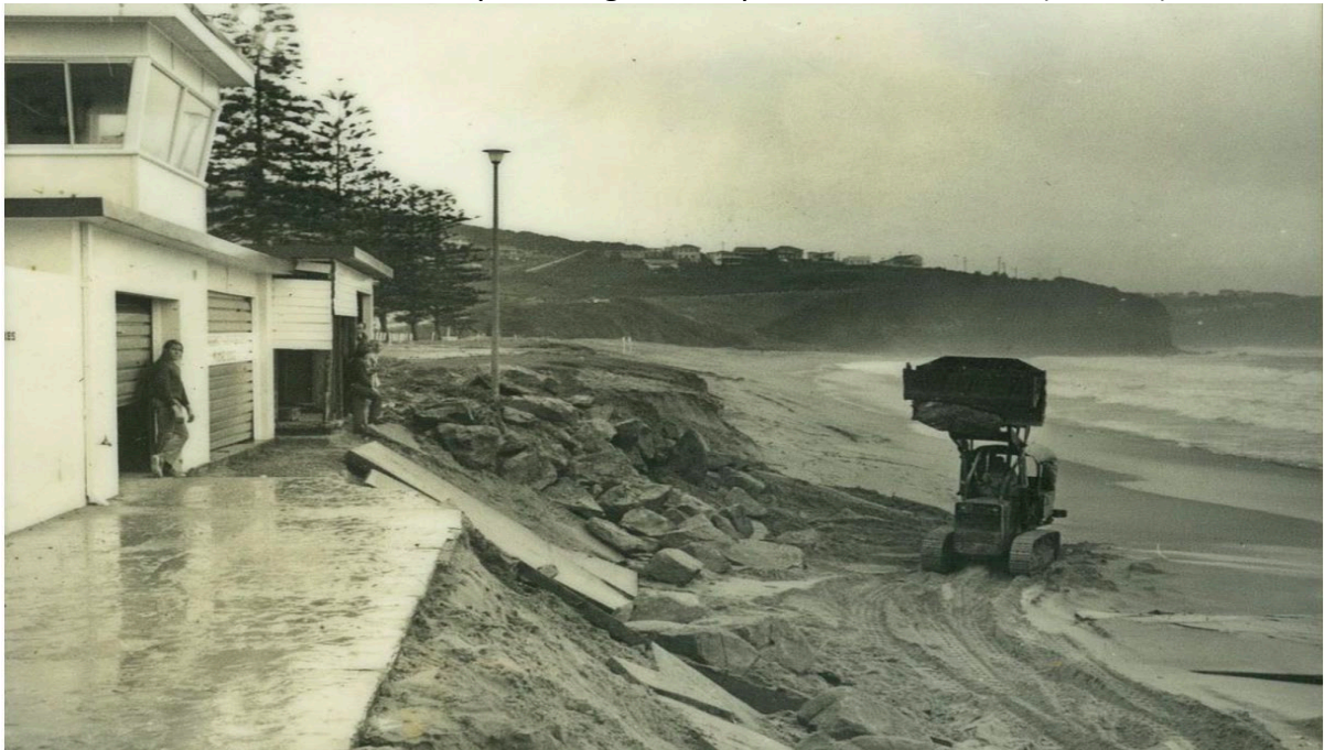
Figure 5: Rock revetment being placed seaward of Newport SLSC on 28 May 1974
