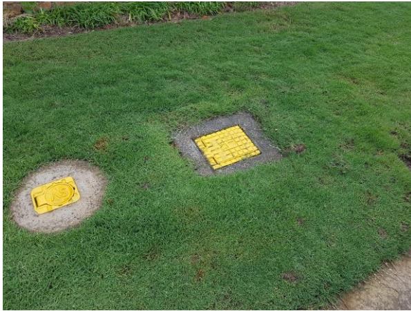
Reticulated water / hydrant in pathway
