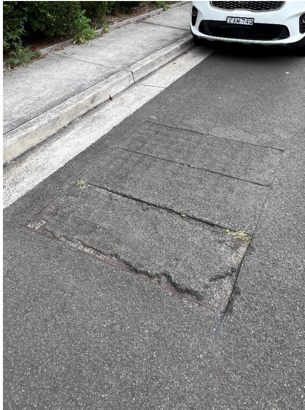
Figure 53 – Crack is evident to the road along the driveway at 4 Pheasant Place, Warriewood.
