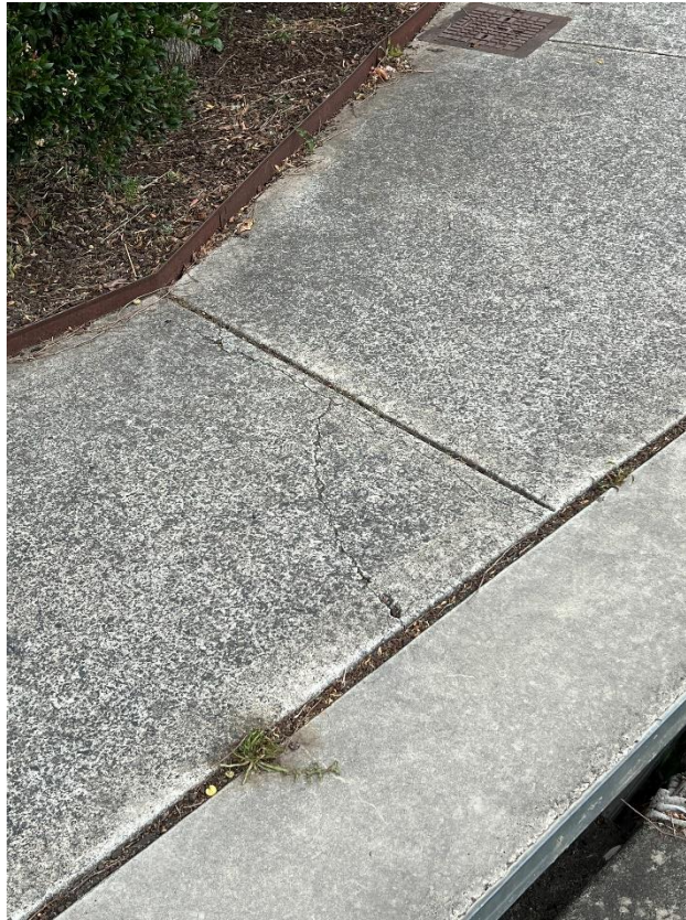
Figure 63 – Crack is evident to the footpath along the driveway at 4 Pheasant Place, Warriewood.
