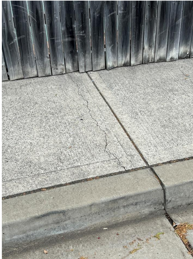
Figure 29 – Crack is evident to the footpath between 14 & 12 Pheasant Place, Warriewood.
