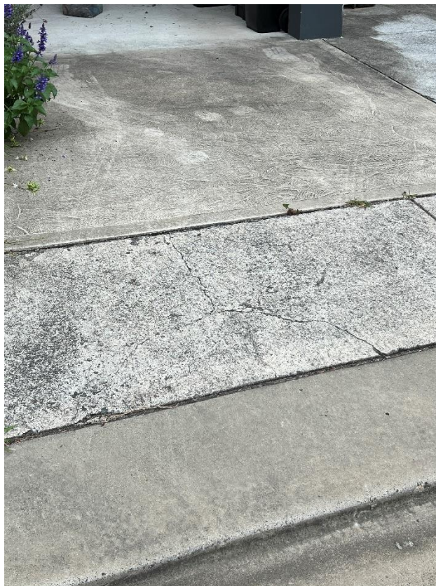
Figure 46 – Crack is evident to the driveway/lapback inside driveway at 8 Pheasant Place, Warriewood.
