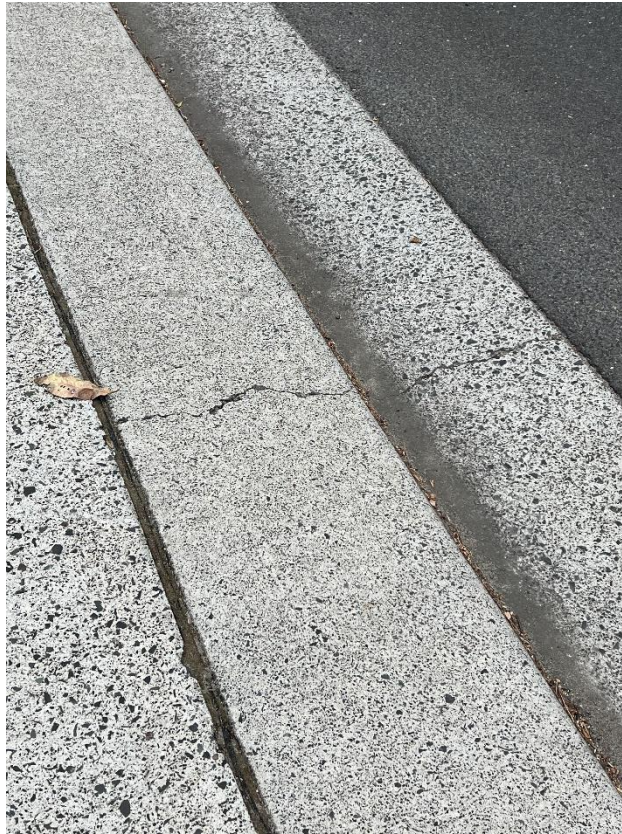
Figure 3 – Crack is evident to the layback to the outside 85 Pheasant Place, Warriewood.
