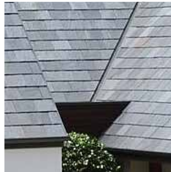
SLATE ROOF NULOK Welsh Slate or similar
