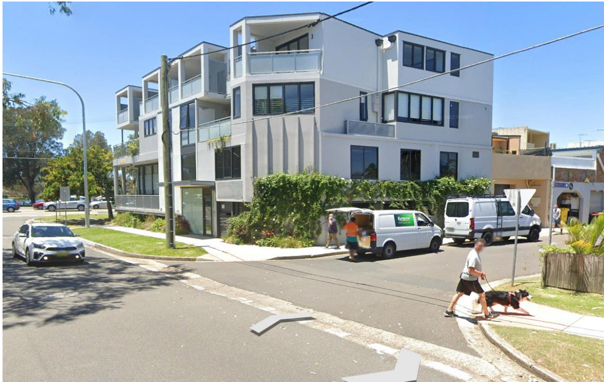
Figure 6 – Shop top housing development to the east 1473 Pittwater Road
