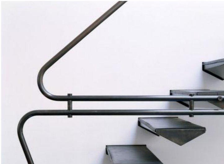
STW 1 STEELWORK - HANDRAIL FINISH SIM/EQ TO DULUX POWDERCOAT 'EARTHEN POT'
