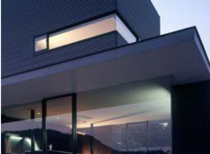
AWN 1 AWNING ALUMINIUM FASCIA COLOUR SIM/EQ TO DULUX 'EARTHEN POT' AWNING SOFFIT IN FC SHEET PAINT FINISH DULUX 'NARROW NECK'
