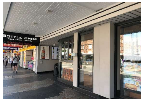
Figure 30 - Ground level shopfront to the Hotel is a later addition, and is generally constructed of powder coated aluminium framing.
