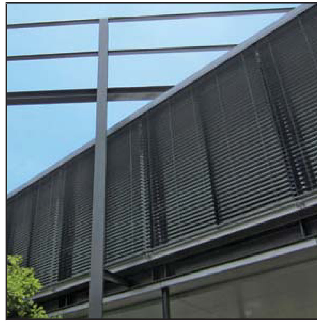
EXAMPLES OF SUN PROTECTION SCREENS: ALUMINIUM LOUVRES COLOUR VARIES VERTICAL AND HORIZONTAL/FIXED AND OPERABLE
