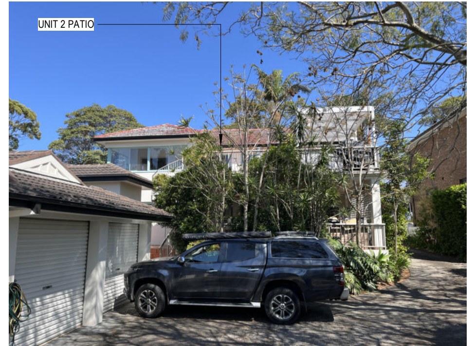
VIEW OF THE REAR OF UNITS 1 & 2
