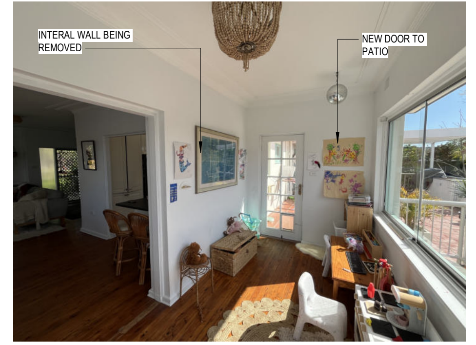
INTERNAL VIEW OF UNIT 2
