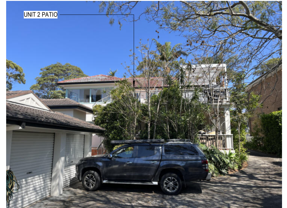
VIEW OF THE REAR OF UNITS 1 & 2
