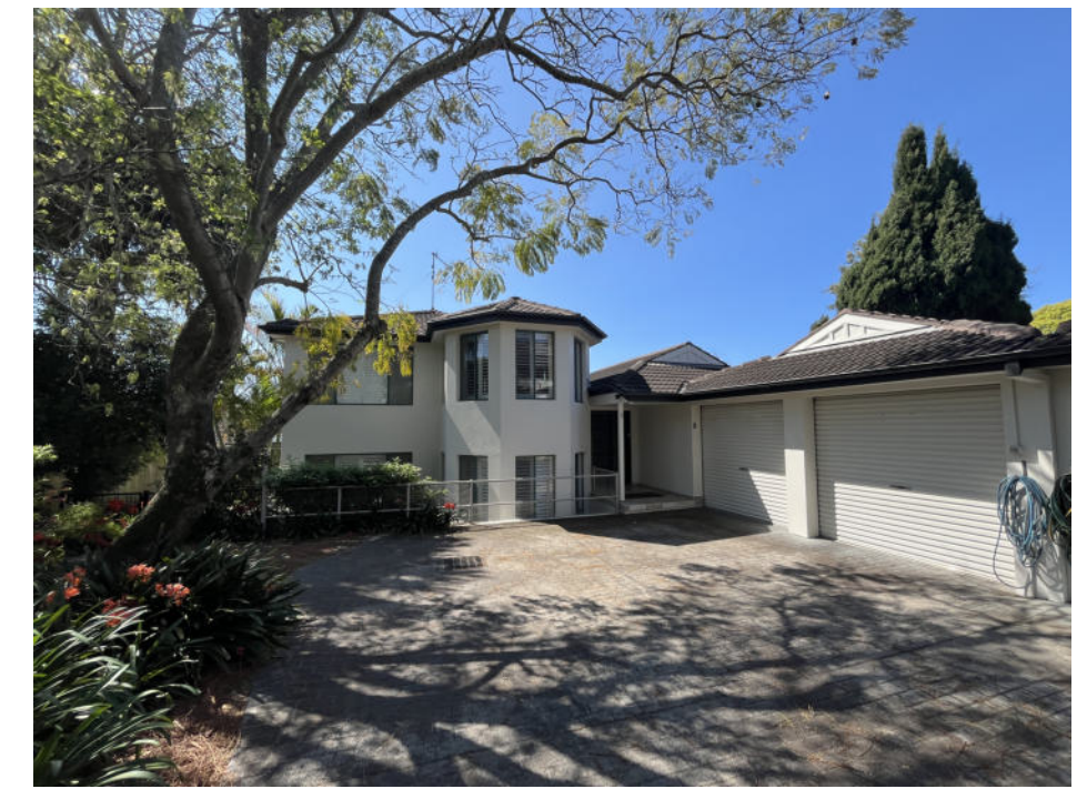
VIEW OF UNIT 3 AT THE REAR OF THE PROPERTY
