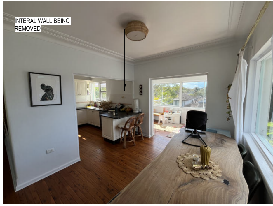
INTERNAL VIEW OF UNIT 2
