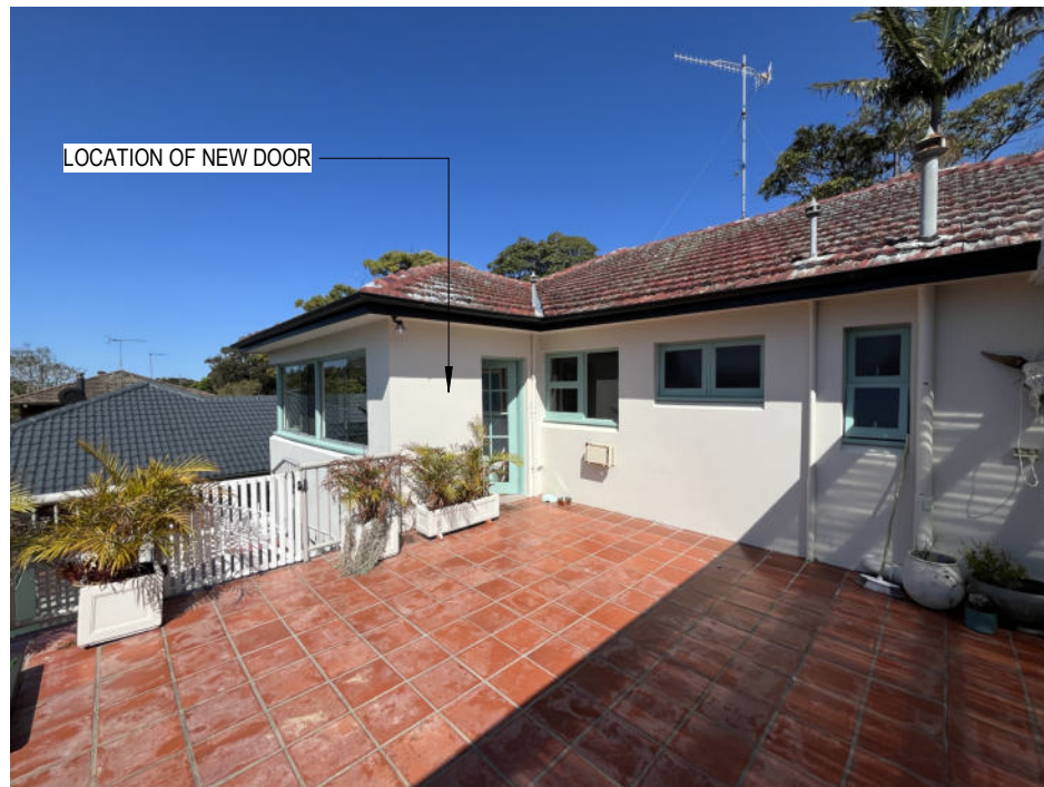
VIEW UNIT 2 PATIO
