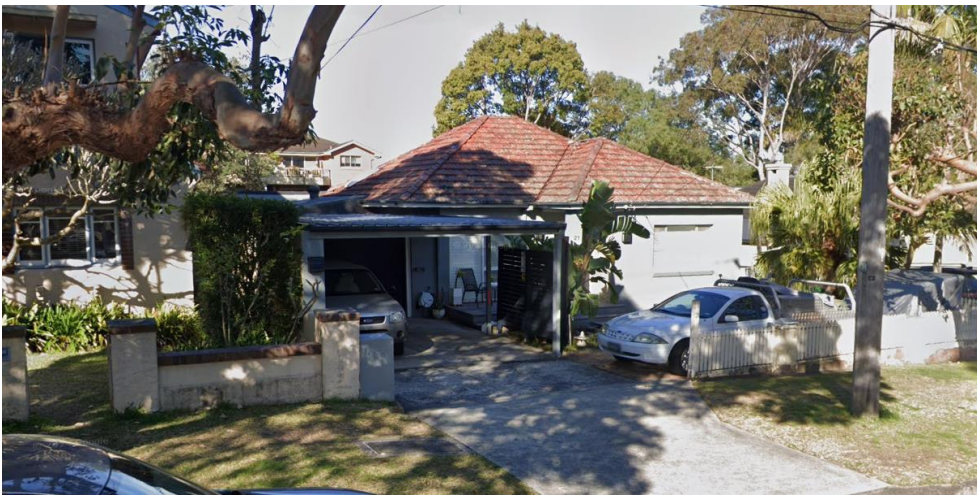
Figure 16. Carport at 21 Innes Road.
