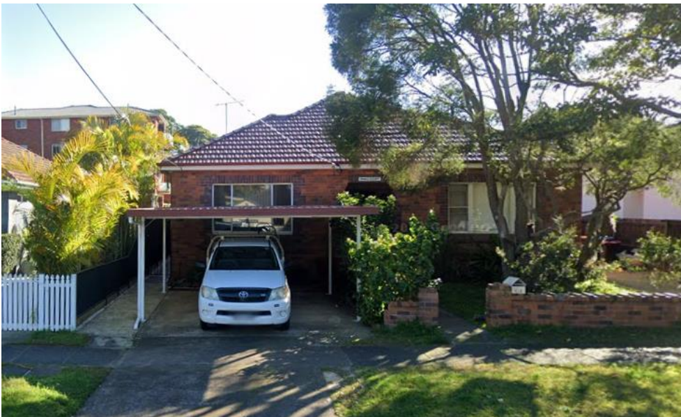
Figure 17. Carport at 28 Innes Road.
