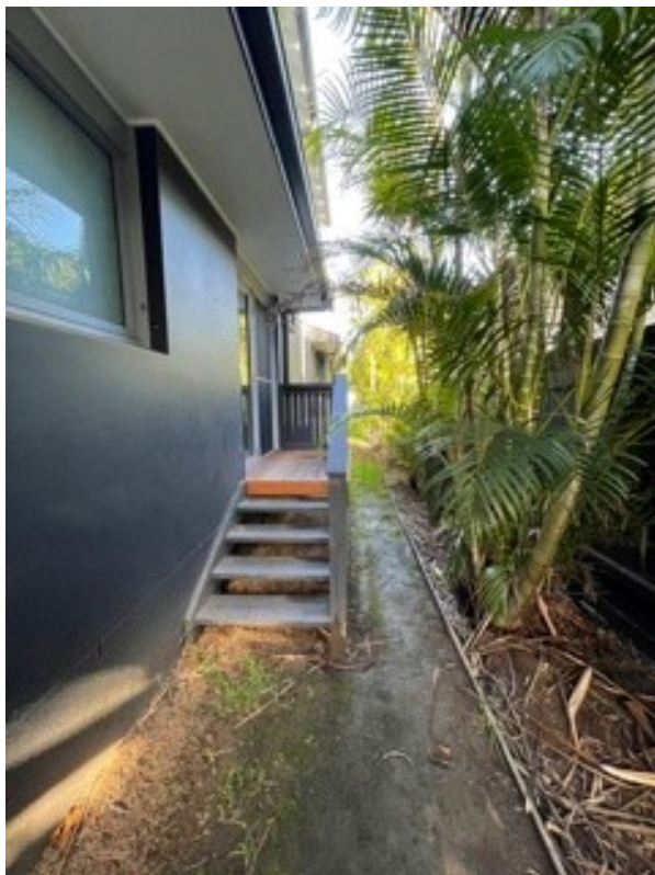
The additional stair and landing to the changed glazed door, to the north side ground floor.
