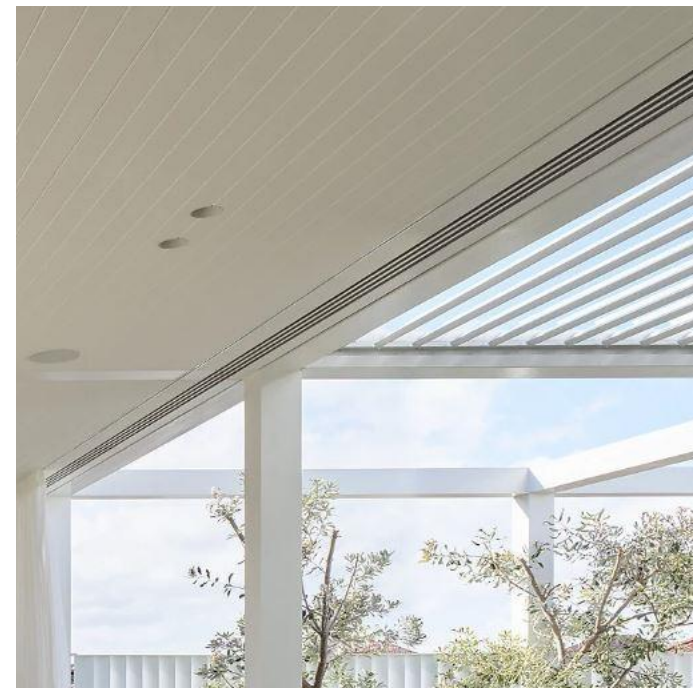
MR METAL PERGOLA STRUCTURE (ABOVE SECOND FLOOR BALCONIES)
