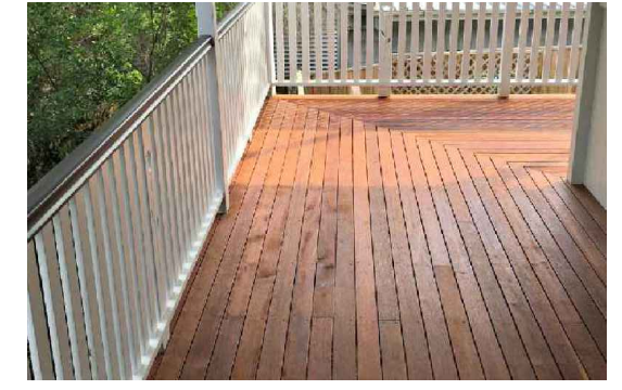
(A) DECK AND BALUSTRADE COMPOSITE DECKING BOARDS WITH POWDER COATED ALUMINUM BALUSTRADE OR SIMILAR TO MATCH EXISTING. COLOUR TO BE DARK AND EARTHY TONED AS PER DCP REQUIREMENTS.
