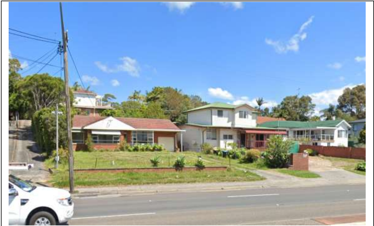
Figure 2.3 – Site and Existing Dwellings Viewed from Warringah Road East to West
