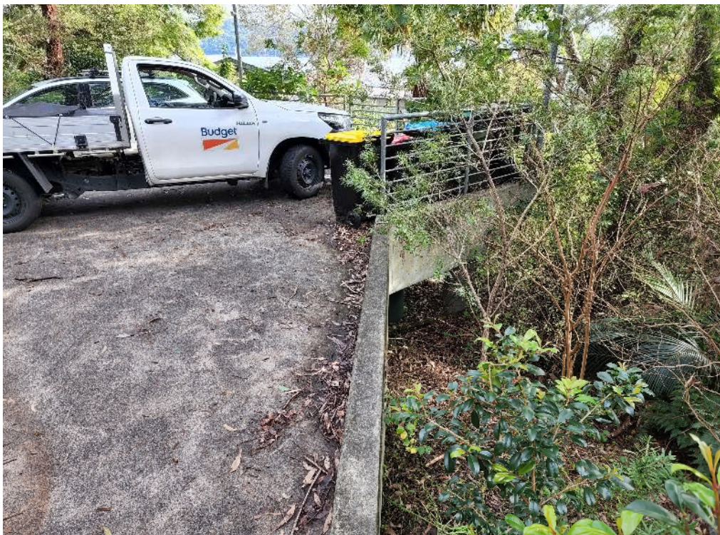
Photo 2: Suspended concrete platform
