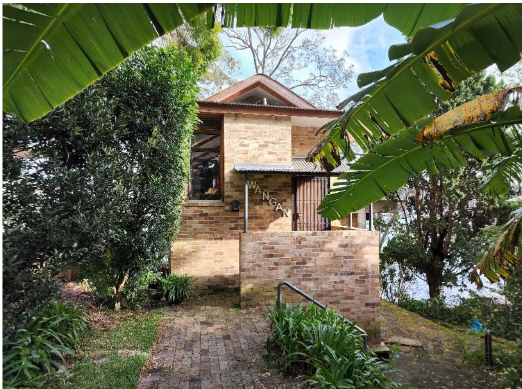
Photo 4: Existing two and three level brick house
