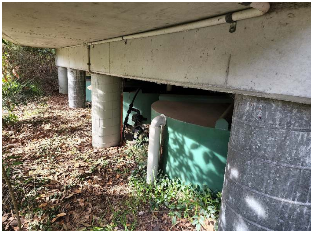
Photo 3: Columns supporting the concrete platform
