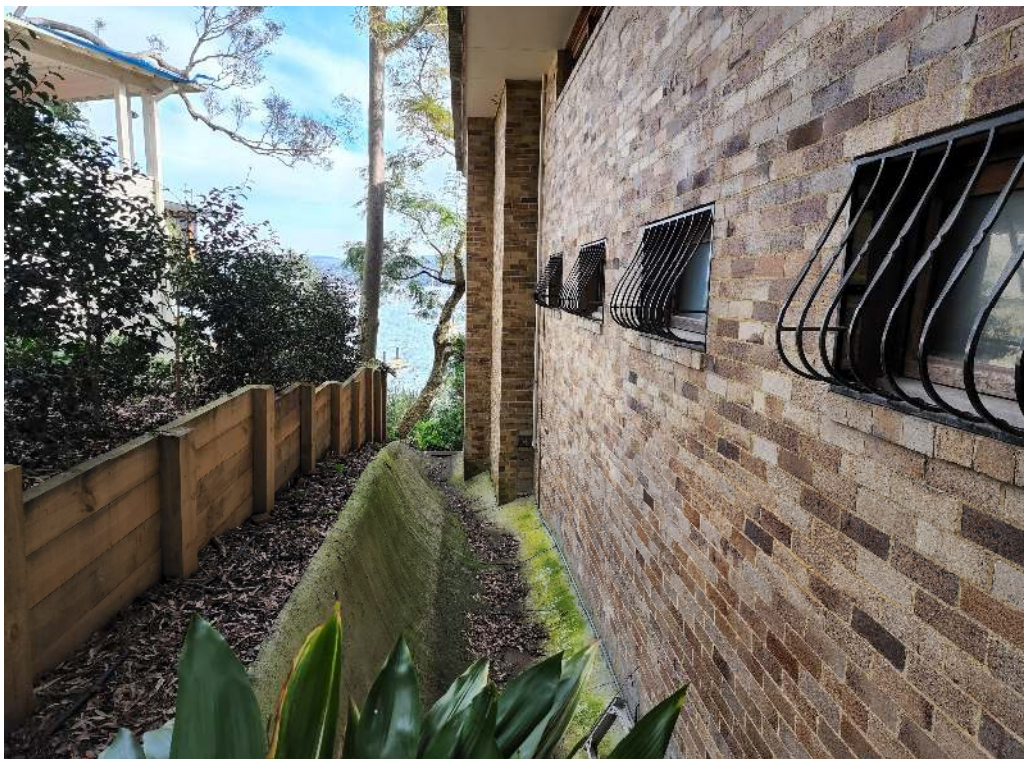
Photo 5: Concrete dish drain along the southern side of house
