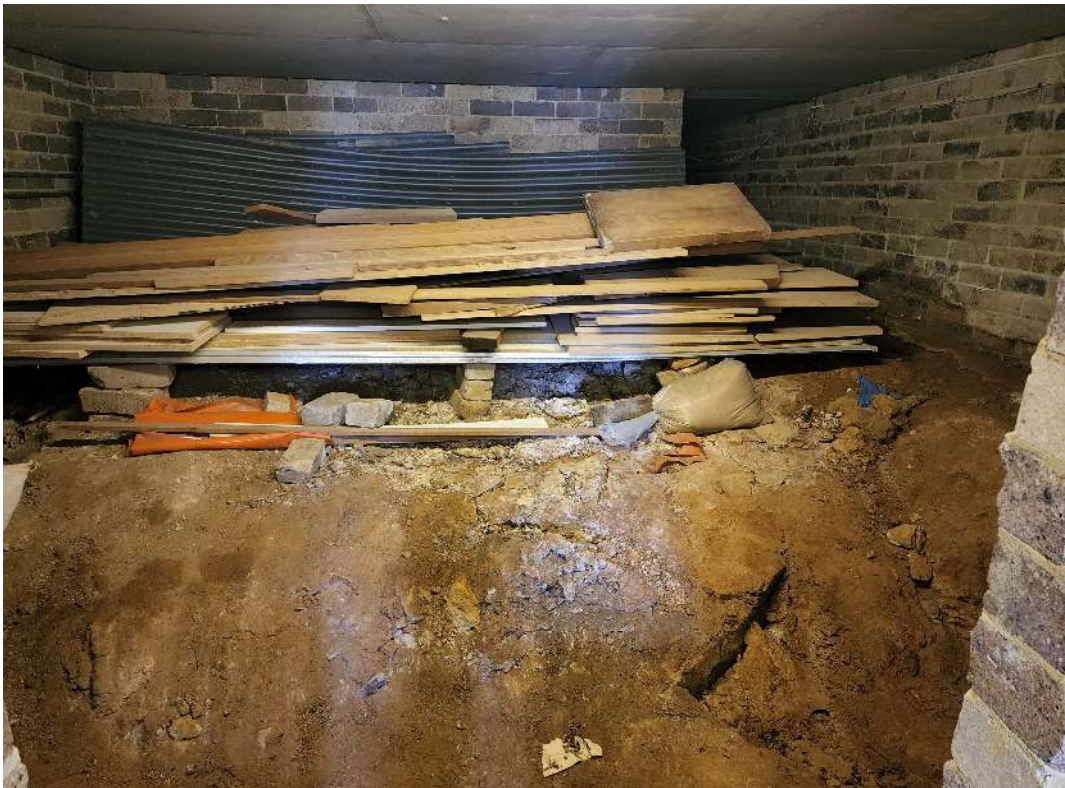
Photo 6: The subfloor of the existing house
