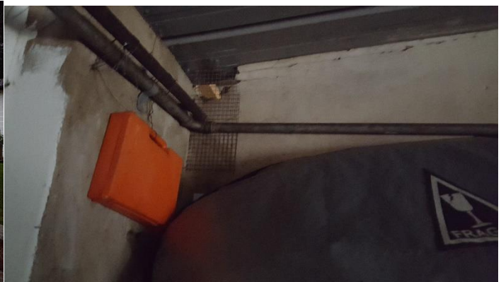
Mesh covering pigeon hole in garage dividing wall
