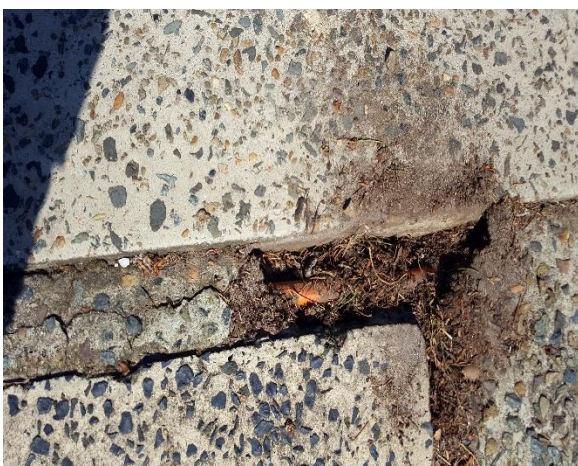
Exposed Electrical Conduit on ROW
