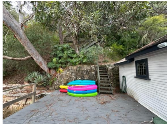
Photo 4: Looking east at the subject site from the jetty and boatshed at the western boundary
