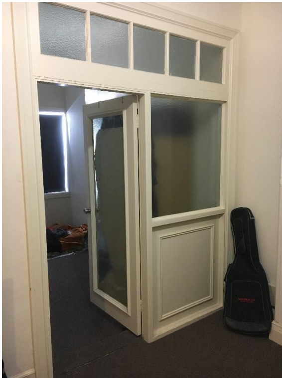
Figure 26: Second floor north unit with early but modified door detailing of the former porch entry.
