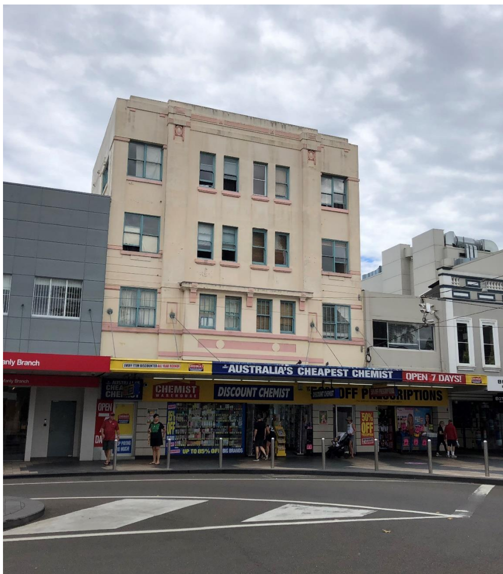
Figure 17 - General view of the main elevation of 19-21 The Corso, showing the varied architectural character of the north side of The Corso.
