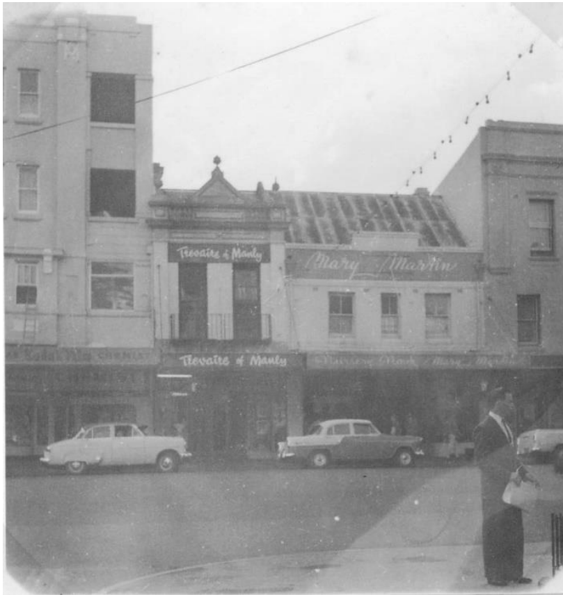
Figure 12 – Photograph said to be dated c1960s, showing 'Exeter Flats' on left, adjacent to Trevaire's at 23 The Corso. (Source: Manly Library Local Studies, File 009642)
