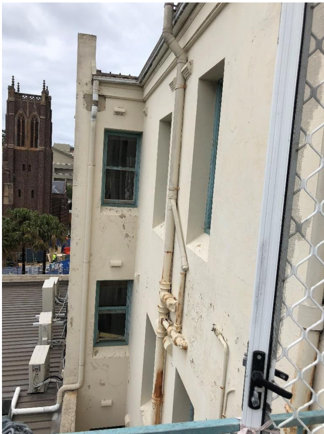
Figure 23: View across lightwell on north-east side of the building.
