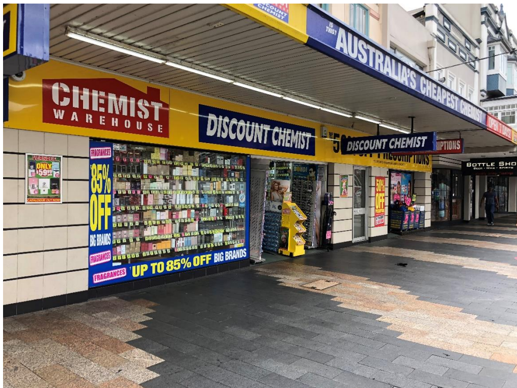
Figure 21: Contemporary shopfronts at ground floor level to The Corso.
