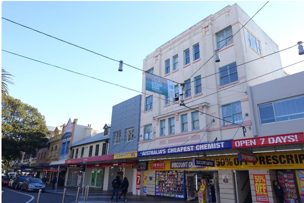
Figure 28 - View of 19-21 The Corso, looking westwards.
