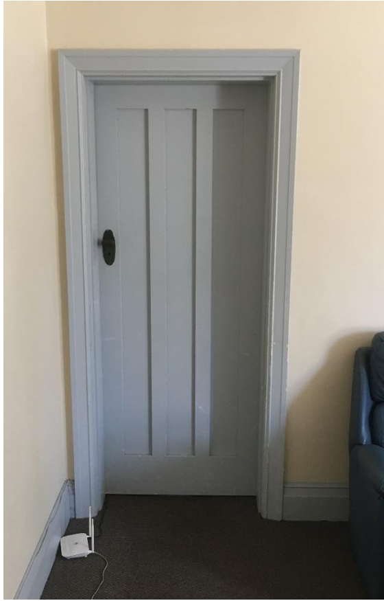
Figure 25: First floor south unit with original door detailing. Note splayed skirting on left side of the photograph.
