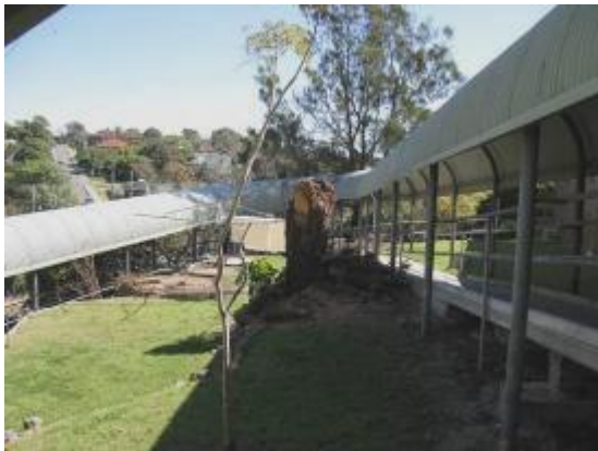
Figure 80: Walkways in front of the Macquarie wing.
