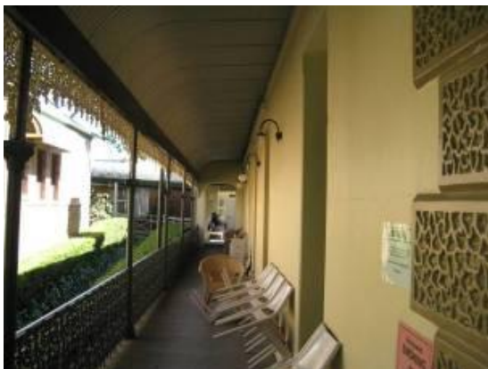
Figure 85: South verandah showing quoins.
