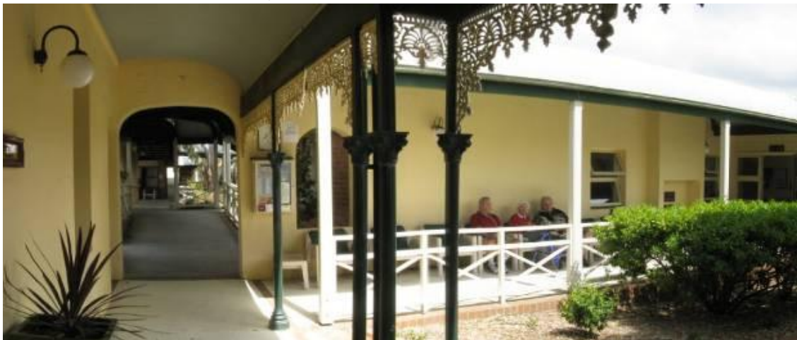
Figure 90: Remnant west wall from the now demolished outbuilding that was attached to the rear of the Pacific Lodge building which now forms part of the walkway around the buildings.
