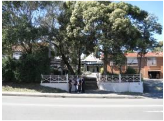
Figure 49: View east to the 1892 Pacific Lodge from Fisher Road.
