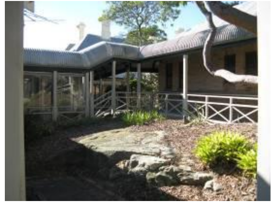
Figure 73: Typical walkways linking the buildings throughout the site. Note also the sandstone outcrop in the foreground and the 1892 Pacific Lodge building to the back.
