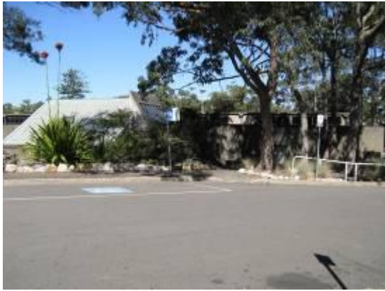
Figure 48: Warringah Library opposite the Pacific Lodge site on Civic Parade. The library is a local heritage item.
