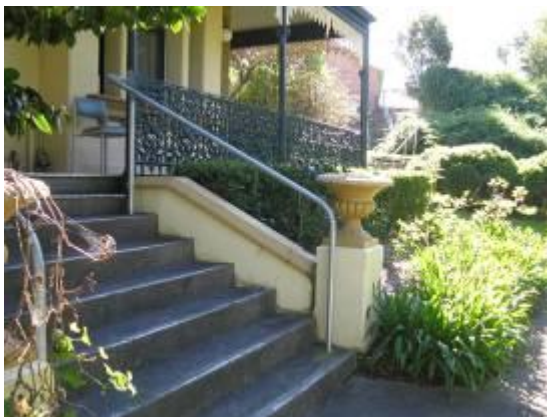
Figure 83: Stairs to the front (east) elevation leading up to the verandah.
