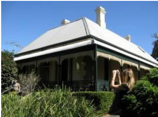
Figure 81: East (front) and north elevations of the Pacific Lodge building.
