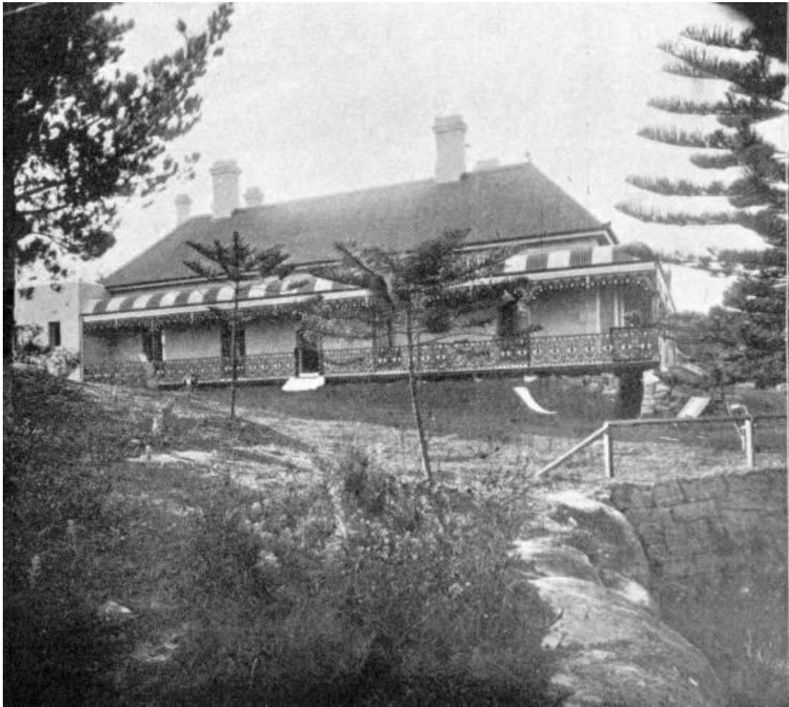
Figure 24: A view of the south elevation of Pacific Lodge, not dated, c.1915. Note the dry packed stone revetment, rock outcrop, and pine tree plantings. Source: Hay, J., Repairers of the breach: a pictorial account of the social work of the Salvation Army throughout the Commonwealth of Australia , Melbourne, 1915.
