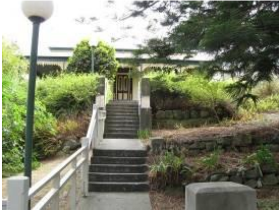
Figure 58: Entry steps and dry stone walls to the front (east) of the 1892 Pacific Lodge building.
