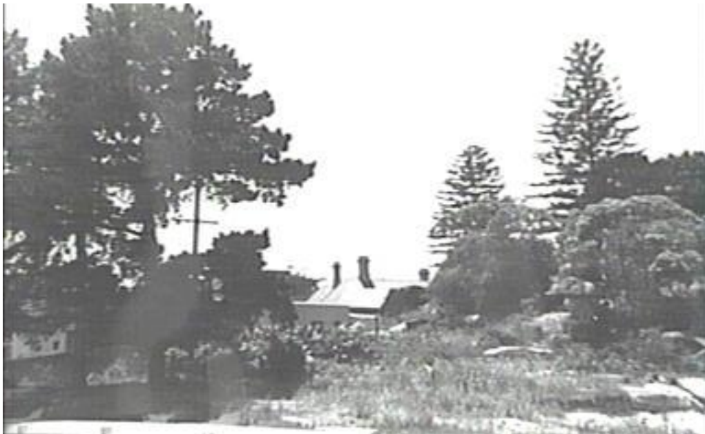
Figure 25: The rear of Pacific Lodge showing the rocky ground and pine trees, not dated, c.1940s. Source: Warringah Library Service Image WAR40097.
