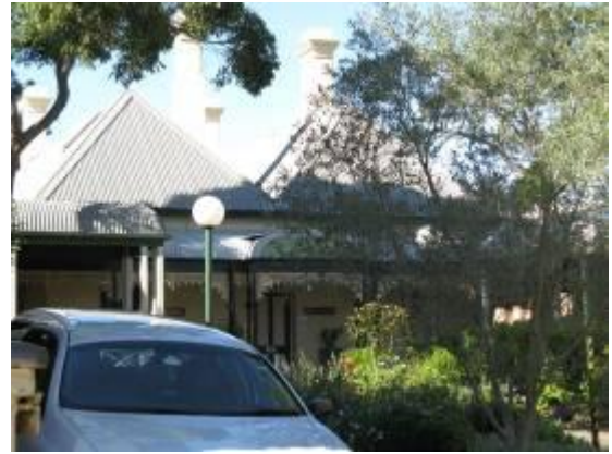
Figure 67: Rear of the 1892 Pacific Lodge building from the west entrance.
