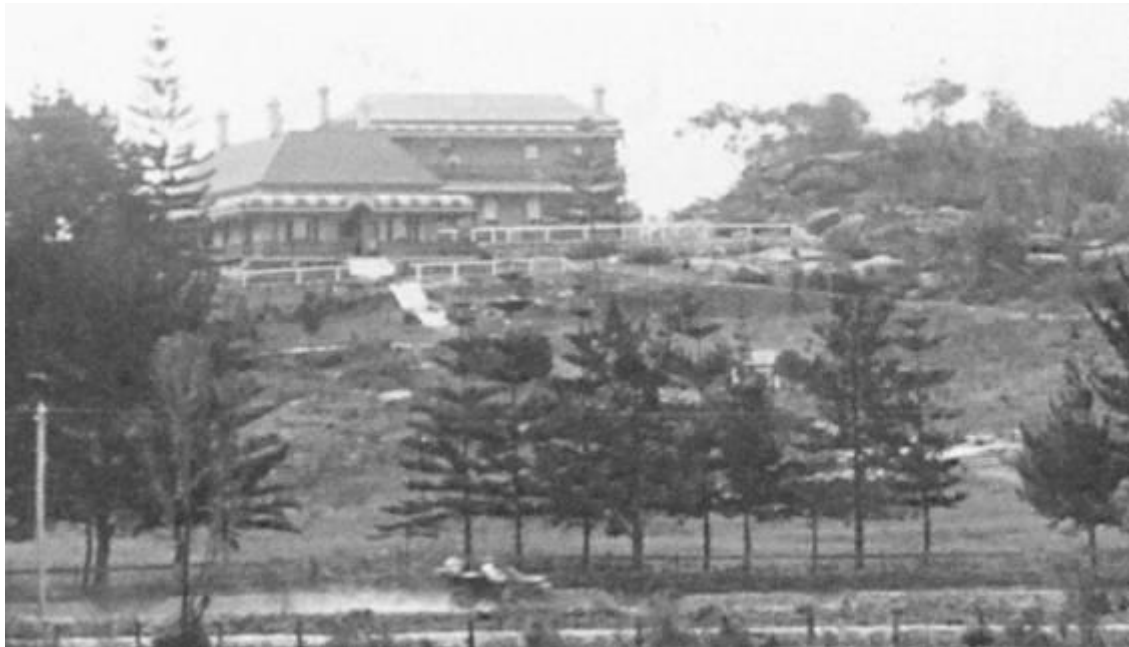
Figure 106: Enlargement of 1912 Image of subject property Source: Warringah Library
