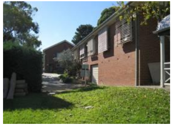
Figure 69: Philip wing (constructed 1992) looking to the Dining Rooms.
