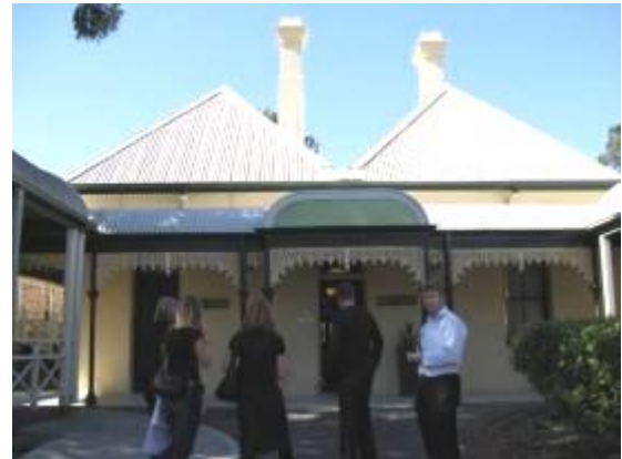
Figure 82: West (rear) elevation of the Pacific Lodge building.
