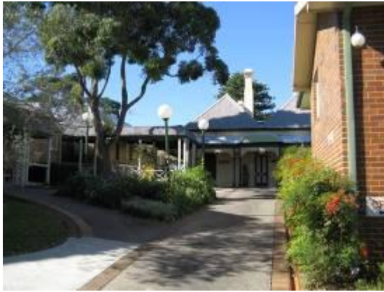
Figure 66: View to the rear of the 1892 Pacific Lodge building from the entry path adjacent the car park.
