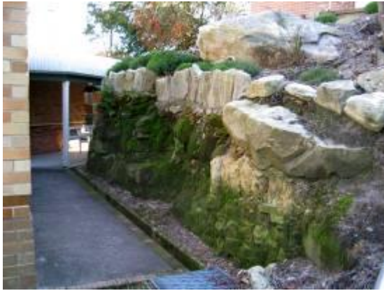
Figure 72: Sandstone outcrop located adjacent the buildings.
