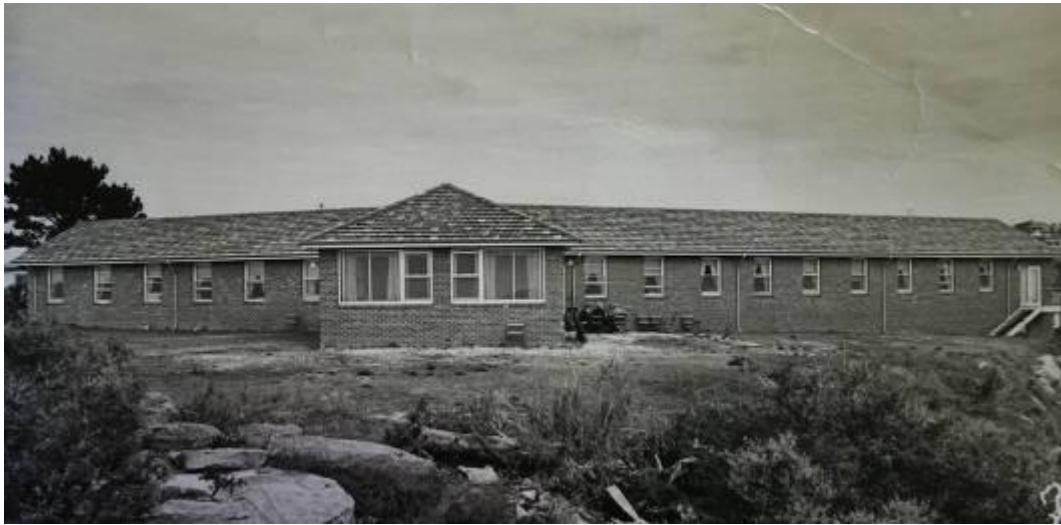
Figure 35: A new accommodation block from the north of the site. Note the rock outcrops. Photograph undated, c1962. Source: Salvation Army Heritage Centre, Booth College, Bexley.
