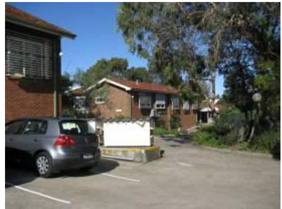
Figure 64: Carpark on the western side of the site off Fisher Road also showing some of the 1962 buildings constructed on the site.
