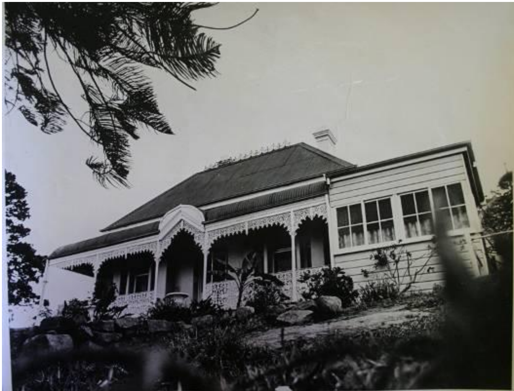
Figure 30: The enclosing of the north verandah was probably undertaken in 1939. Note the sliding sash windows. Photograph date circa early 1960s. Source: Salvation Army Heritage Centre, Booth College, Bexley.
