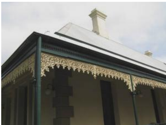
Figure 89: Decorative lace work to the verandah. Note also the tall corbelled chimneys.
