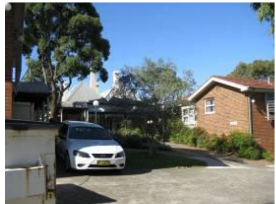
Figure 66: View to the rear of the 1892 Pacific Lodge building from the car park.
