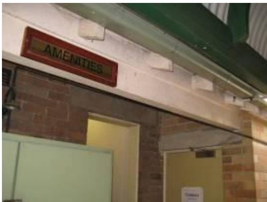
Figure 76: Heritage significant amenities building detail.
