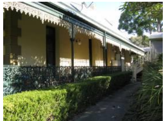
Figure 84: General view of verandah.
