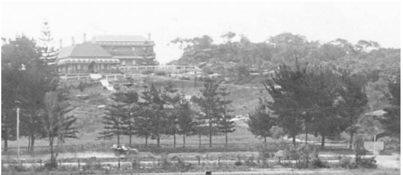
Figure 23: Pacific Lodge, not dated, late 1910s (note the speeding motor car). The photograph depicts the 1892 cottage and 1911 two storey dormitory block as well as landscaping with pine trees within the grounds and along Pittwater Road. Source: A Warringah Library Service Image reproduced in Boyce, J., Pictorial History: Warringah , Kingsclear Books, 2006.
