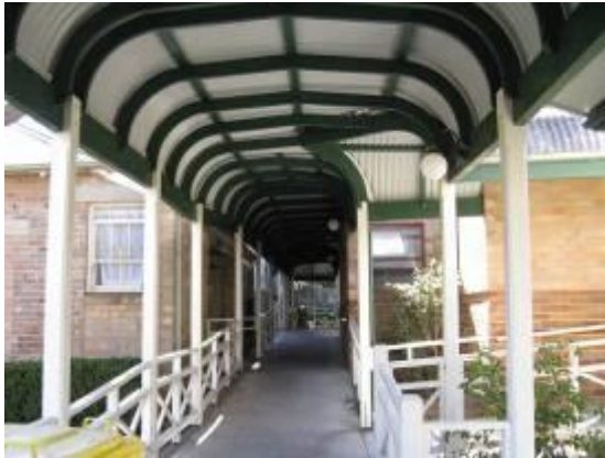
Figure 74: Walkways through the site.
