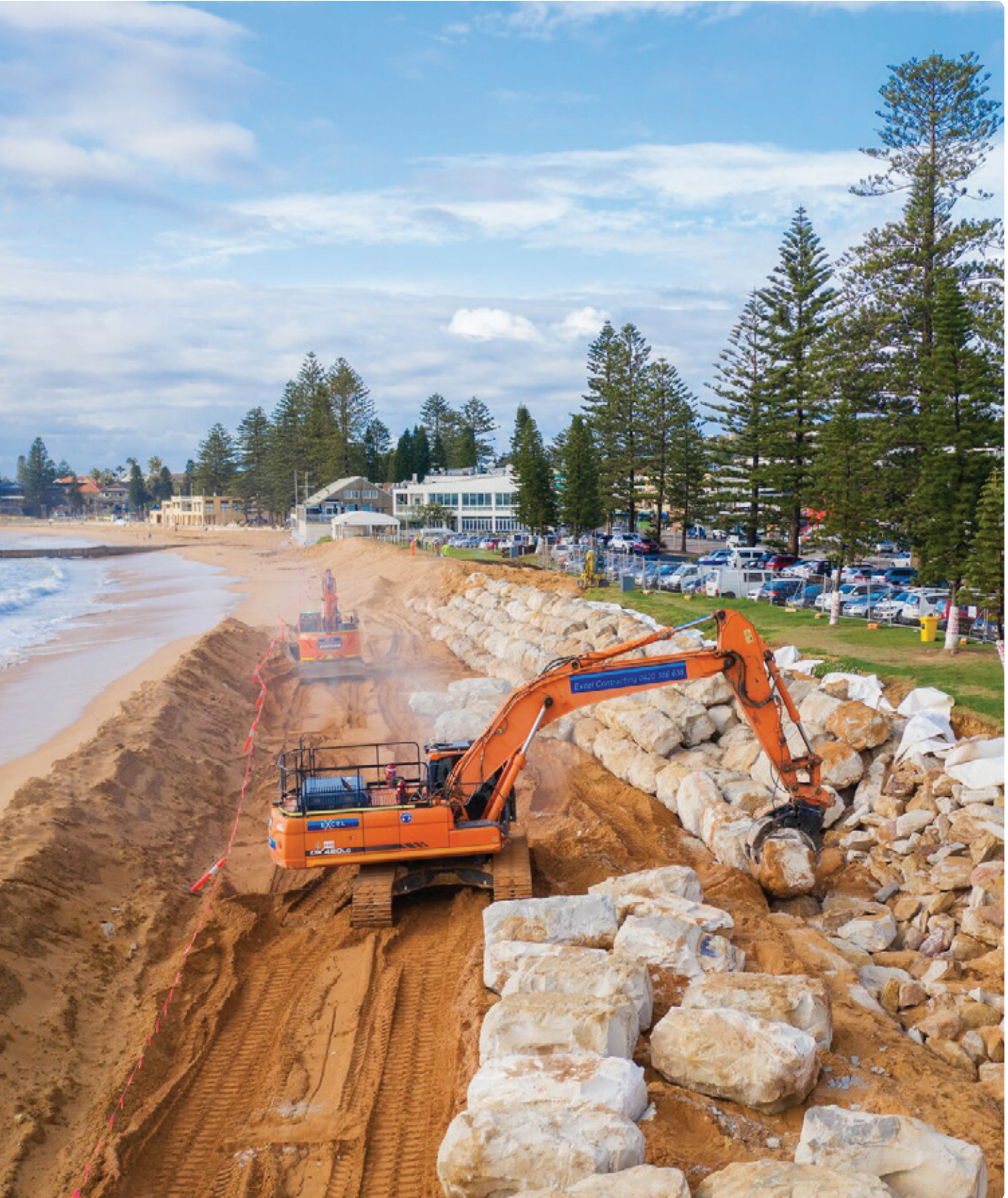
Collaroy Beach seawall
