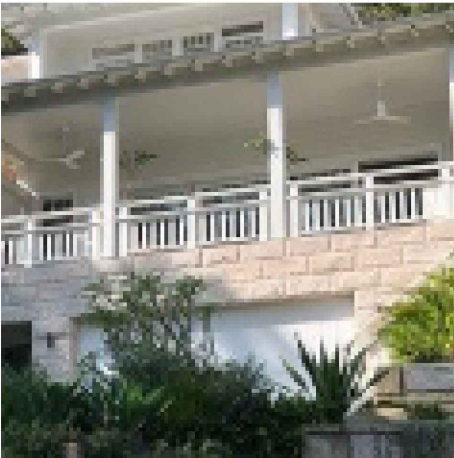
Exterior Sandstone Rockface Cladding to Garage Columns
