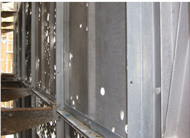
Picture 3 – internal construction of panels Source: Buchan
