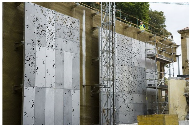
Picture 4 – external construction of panels Source: Buchan
