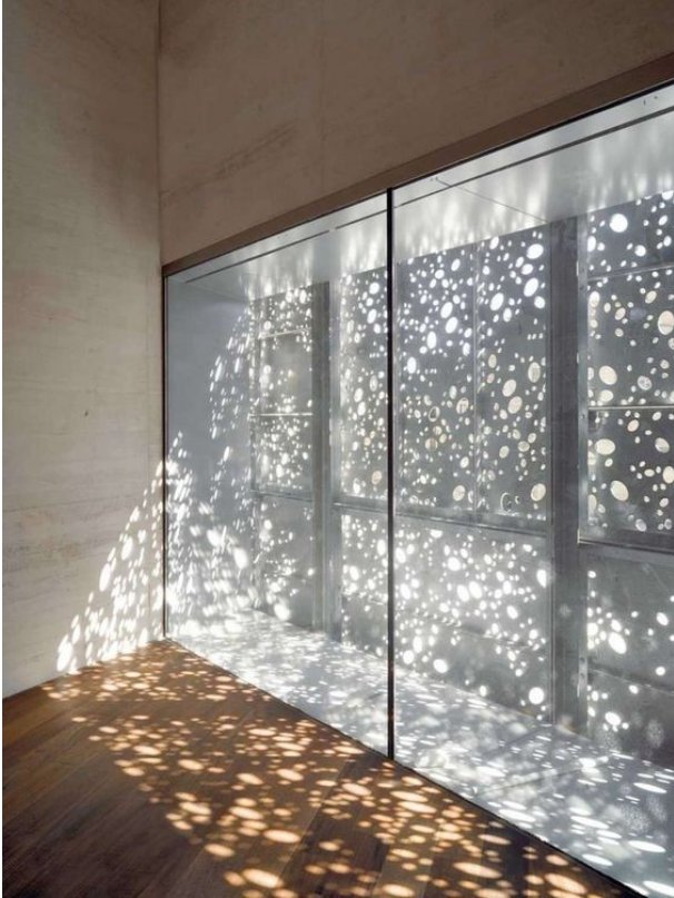
Figure 4 -Sample images relating to the GRC-01 permeable façade material on the Forest Way elevation
