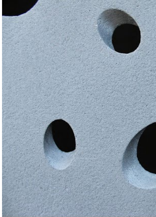
Picture 2 – external facade Source: Buchan
