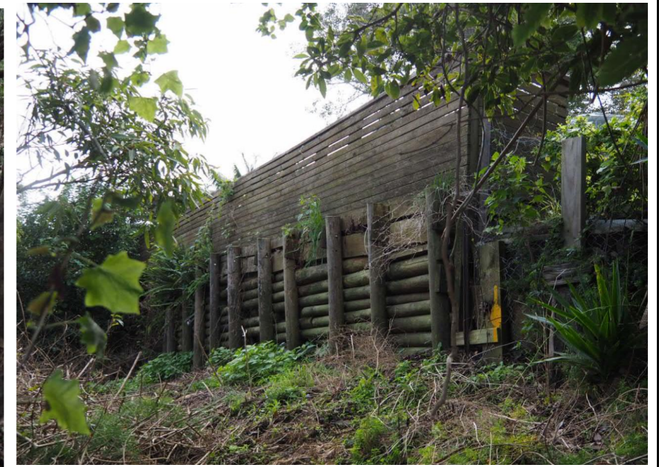
Photo 6: Timber log wall at northern boundary supporting upslope property
