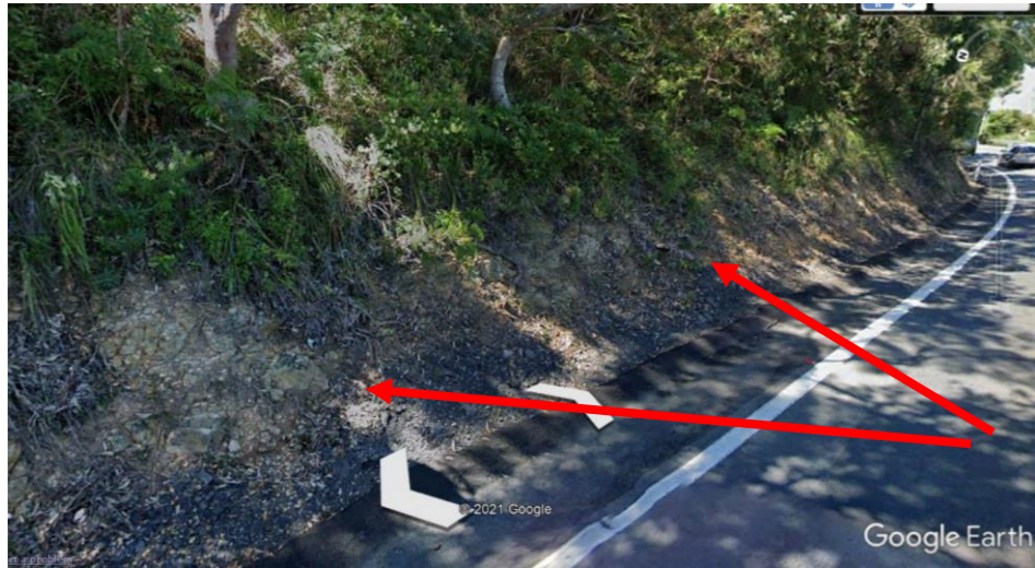
Photo 1: Bedrock exposed in excavated batter alongside Barrenjoey Road. (Google Streetview March 2020)
