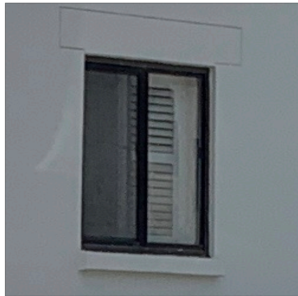
07 DORMER WINDOW FRAME Black frame & fenestrations. Recessed expressions in render to match existing.
