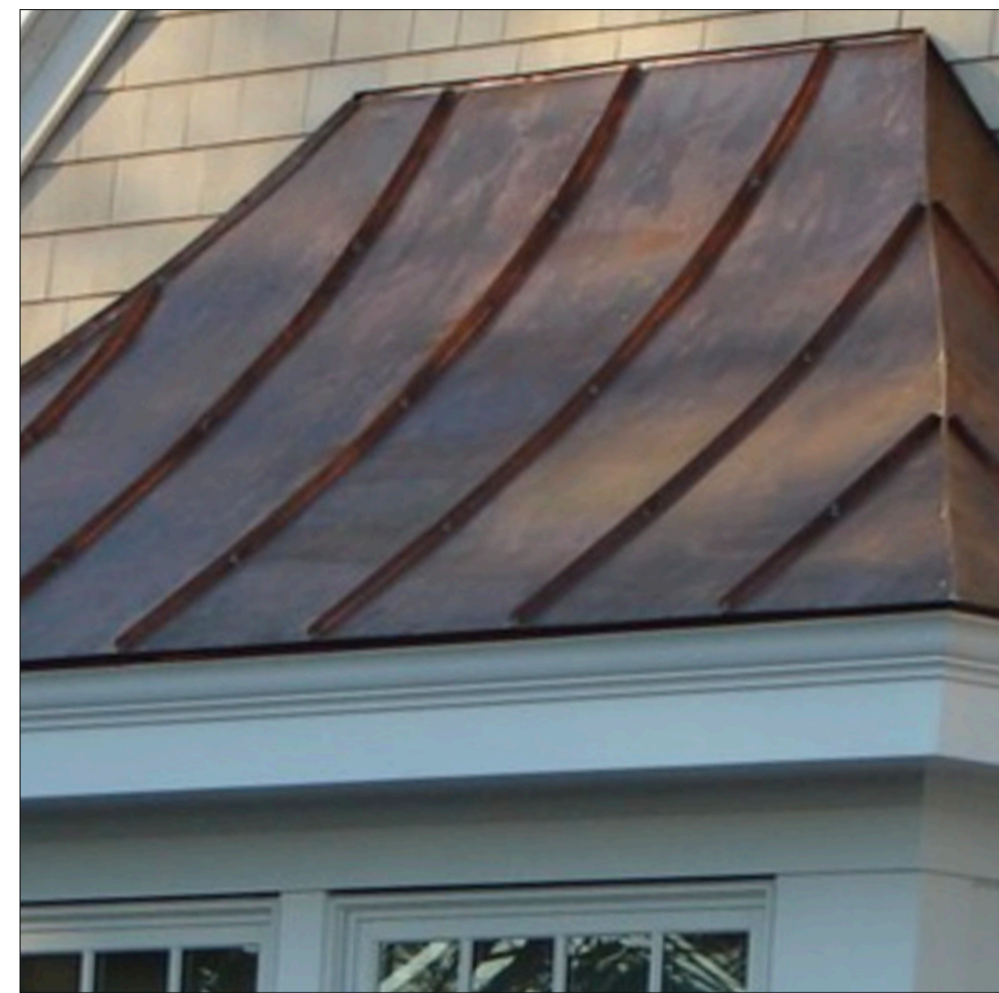
02 DORMER ROOF Aged Copper Standing Seam
