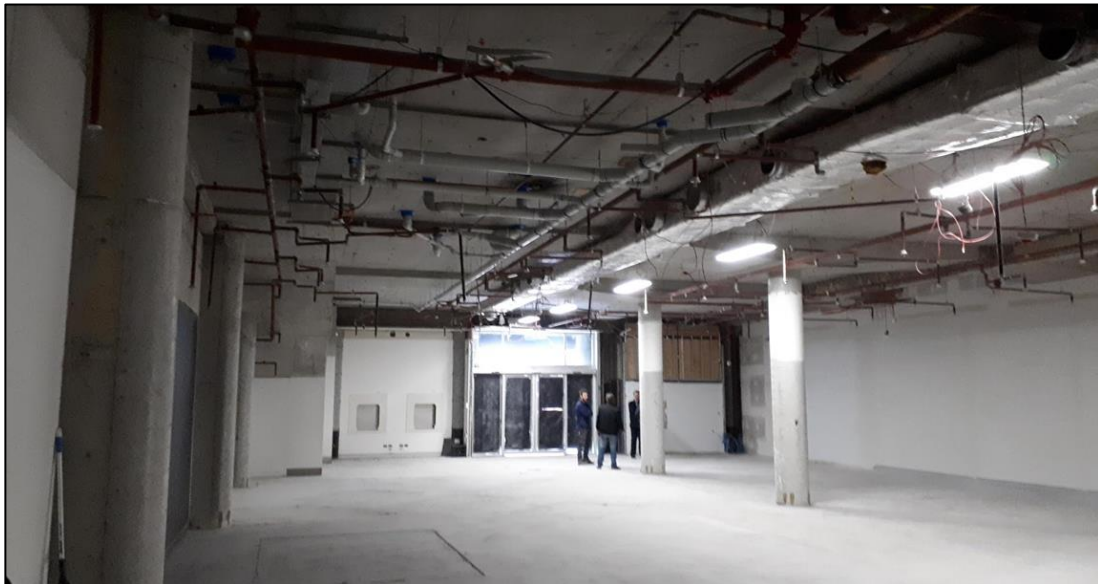
Figure 7. Existing internal ground floor facing north-west Source: Mecone
