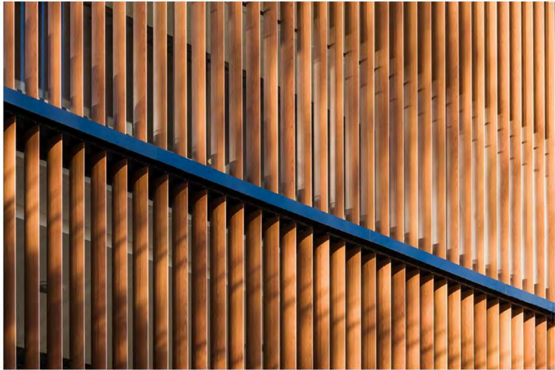
EW-01 VERTICAL LOUVERED GLAZING - TIMBER LOOK
