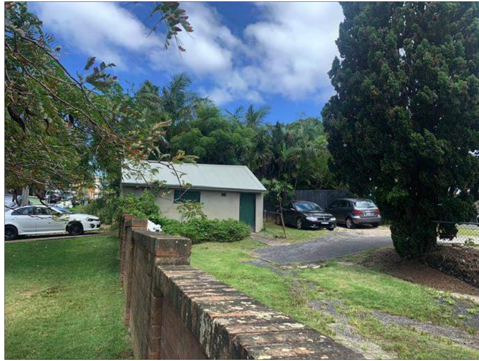
30 OLIVER ST LOOKING FROM DOWLING ST EASTERN BOUNDARY
