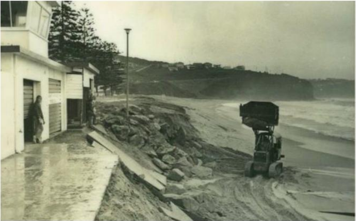
Figure 1.3 Storm damage and emergency works, 28 May 1974 (Horton, 2020)
