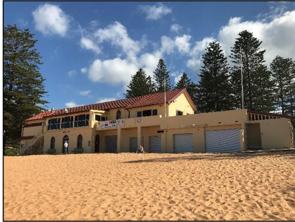
Figure 11. View of the eastern elevation as seen from Newport beach.
