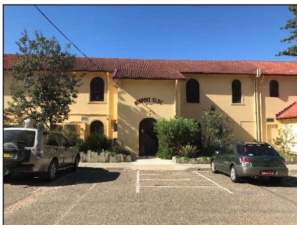
Figure 9. View to the entrance portico along the Western Elevation.
