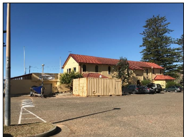
Figure 10. View from the north-western corner of the parking lot looking towards the subject building.
