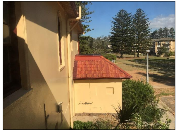
Figure 26. View of the Southern wing as seen from the office above the entry portico.
