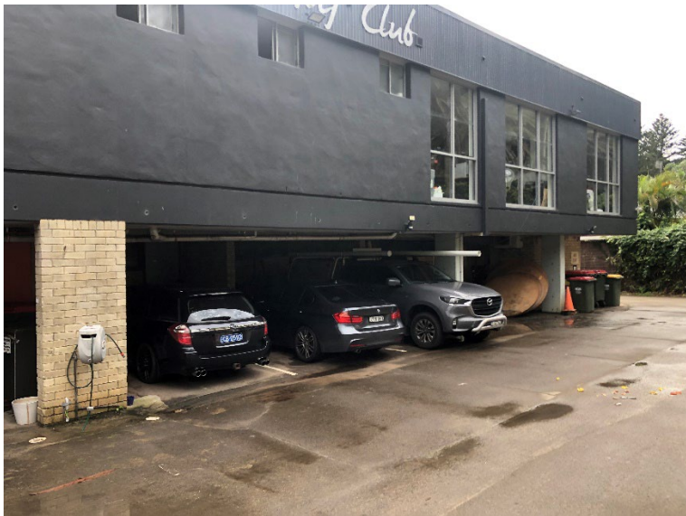
Figure 3. View from rear carpark to south façade of building.
