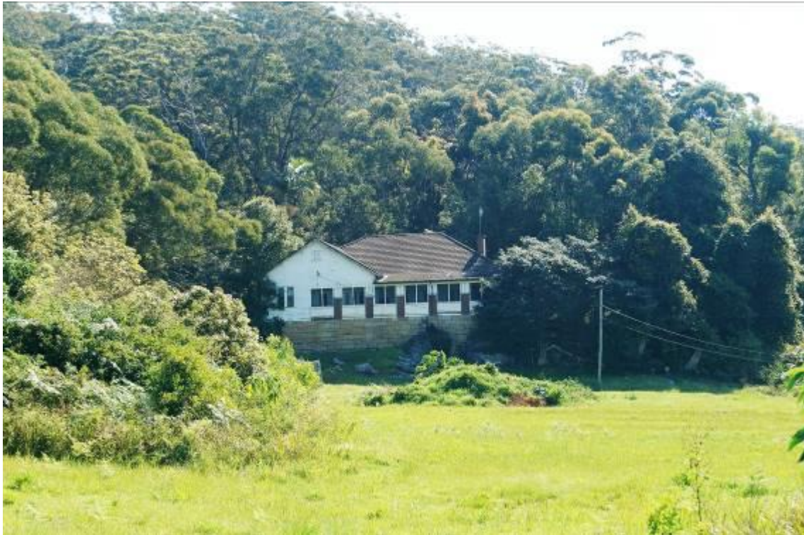
Figure 9 - View looking west from centre of site towards existing dwelling house
