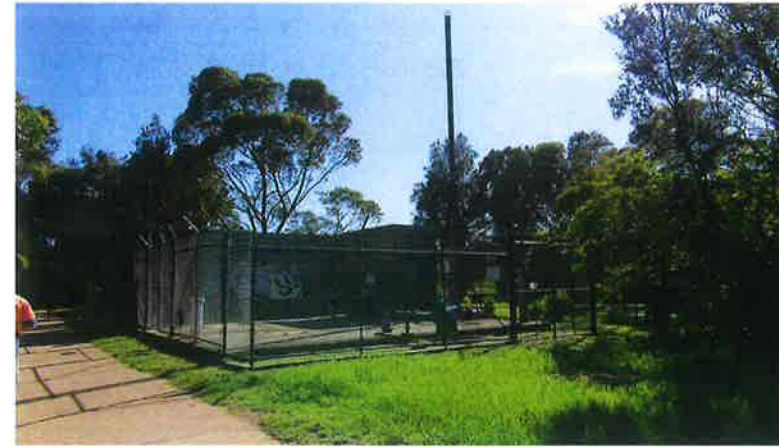
View from point C Direction / North-East Looking at SYD Water Pump out facility Taken from the path 2
