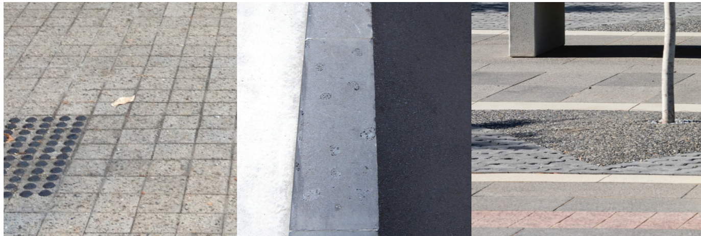
Concrete cobble as robust and durable natural stone alternative
