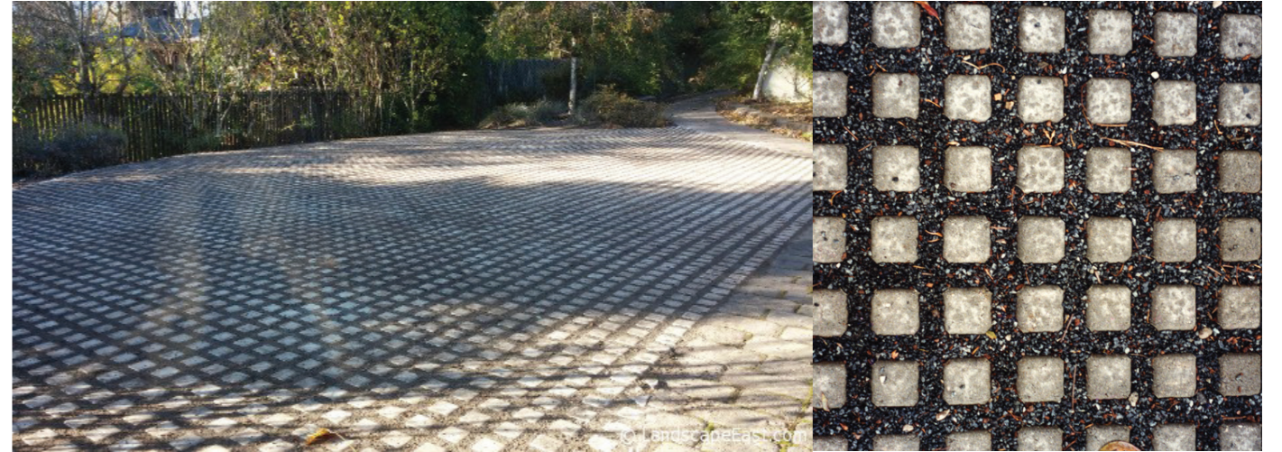
Permeable paving grasscrete for carpark
