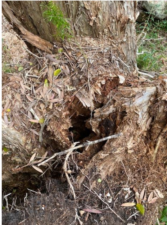
Figure 2: Cavity at base
