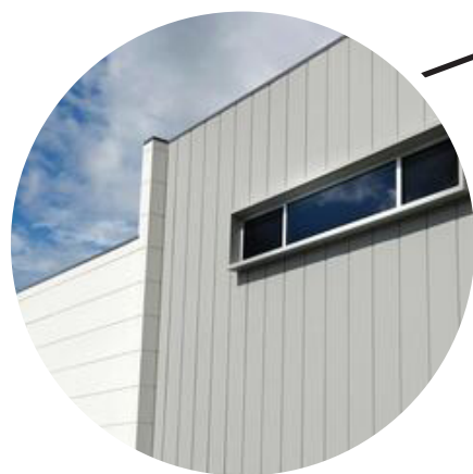
VERTICAL PANEL CLADDING
