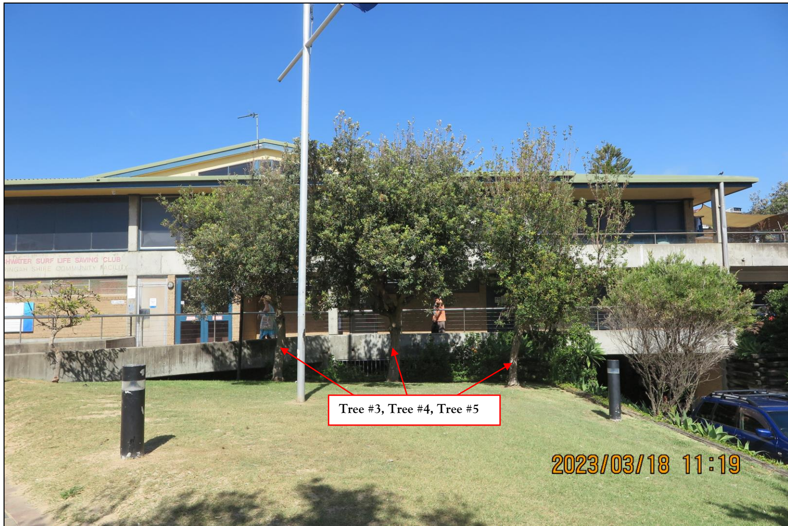
Figure 9: Illustrates the location & condition of Tree 33, Tree #4 & Tree #5.
