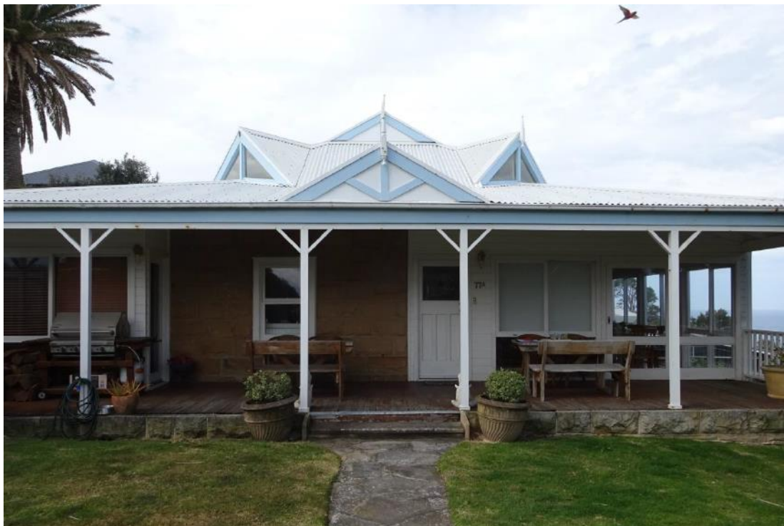
Fig 2: View of subject dwelling, looking south-east
