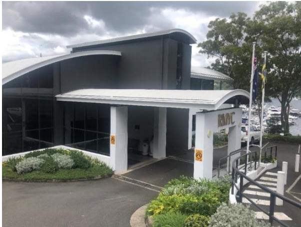
Figure 16 RMYC building viewed from upper carparking area
