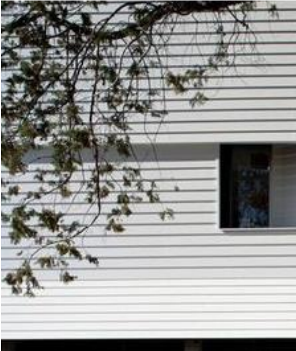
Weatherboard walls for new dwelling
