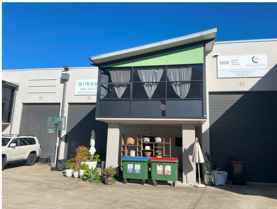
Figure 6 – current premise frontage
