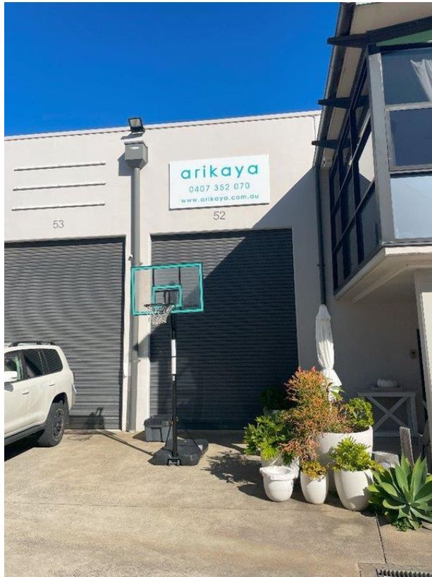
Figure 5 – current premise frontage and signage panel
