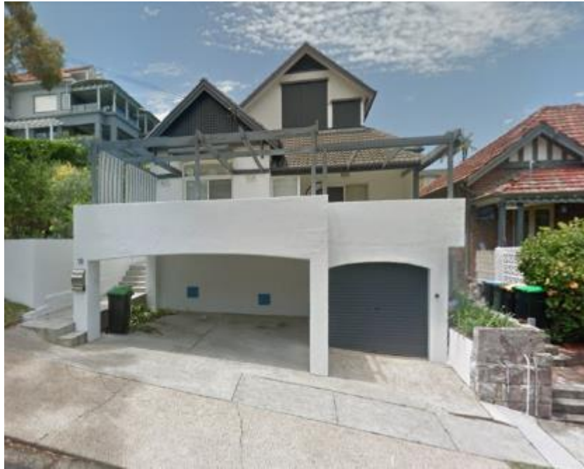
View of Subject Site from Street
