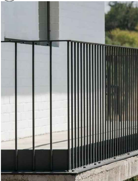
DARK STEEL OR TIMBER BATTEN BALUSTRADE DULUX FERRODOR 810 - NATURAL GREY OR EQU.
