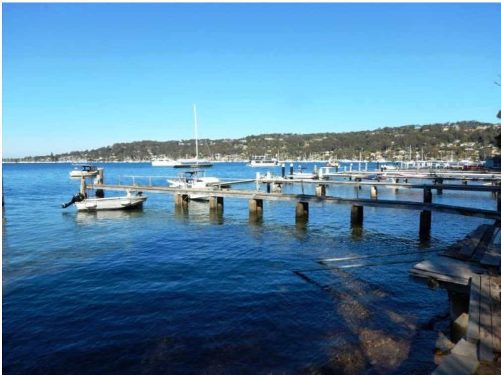
Photo 2. The existing waterfront structures (with slip rails in the foreground) as viewed looking to the south.
