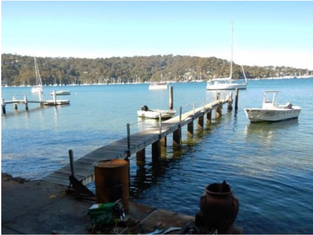
Photo 1. The existing timber jetty and berthing piles at The Property.
