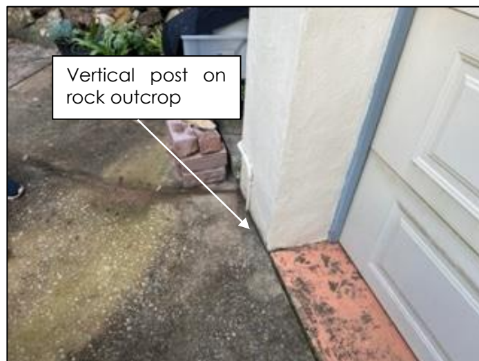
Photo 6: Footing on concrete – top of driveway (left side of house frontage)
