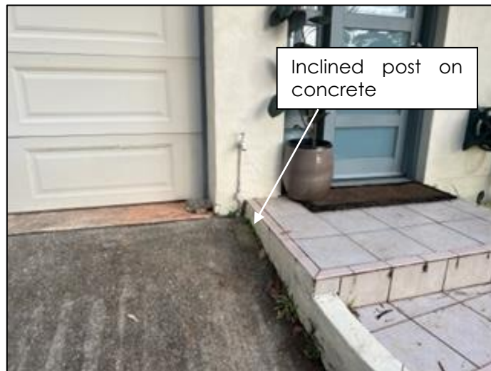
Photo 5: Footings on concrete – top of driveway / stairs
