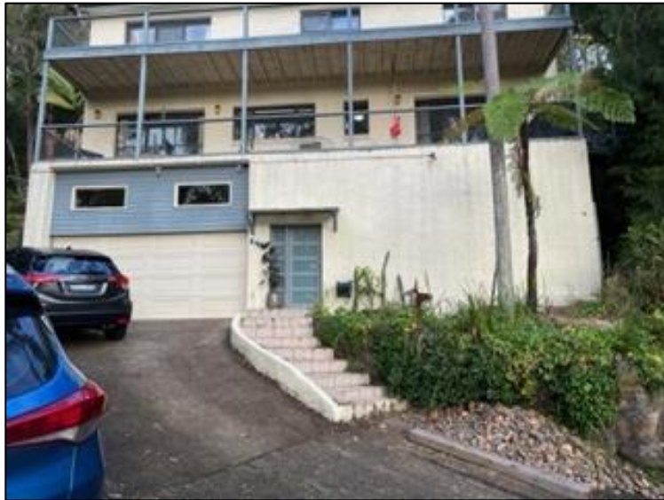
Photo 1: House frontage – concrete driveway and access stairs
