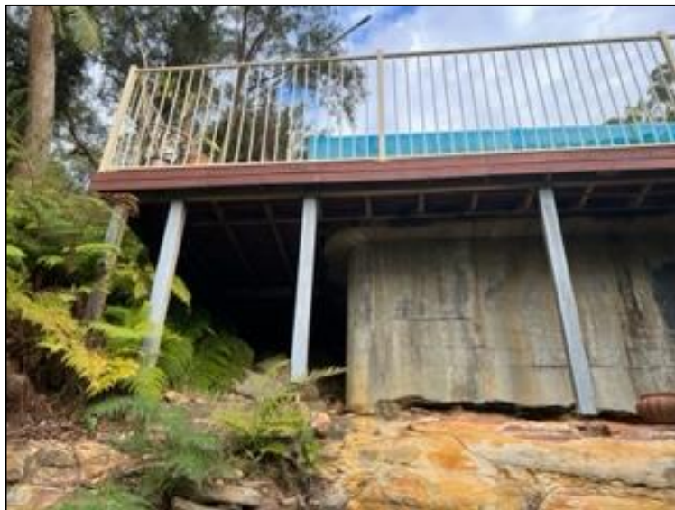
Photo 2: Steel posts supporting the pool
