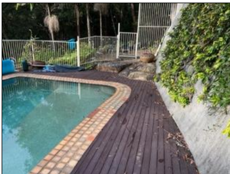
Photo 3: Shotcrete on cut face of pool
