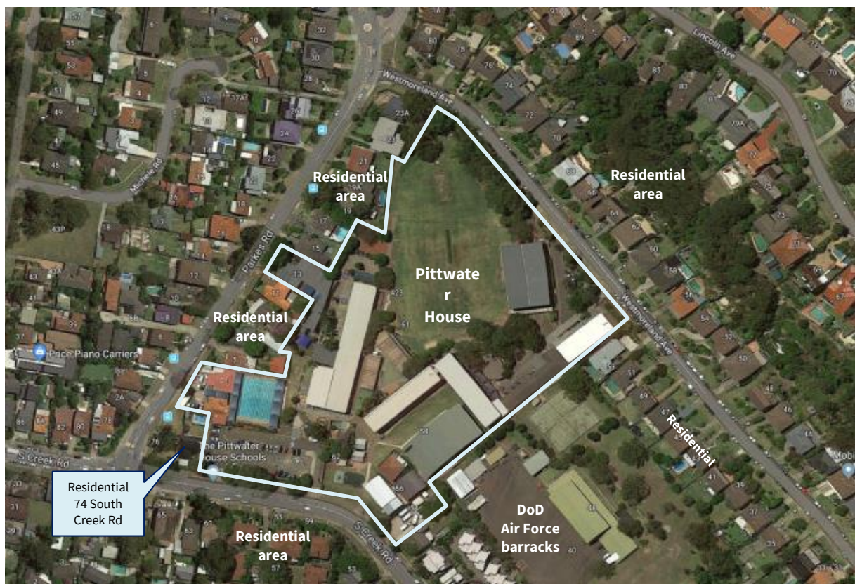
Figure 1. Aerial view of the school and surrounding properties
