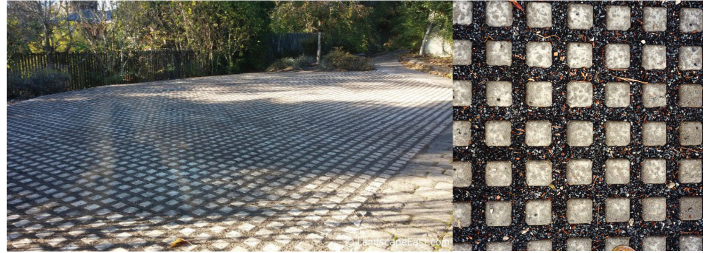
Permeable paving grasscrete for carpark
