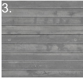
3. WALLS CONCRETE - OFF FORM
